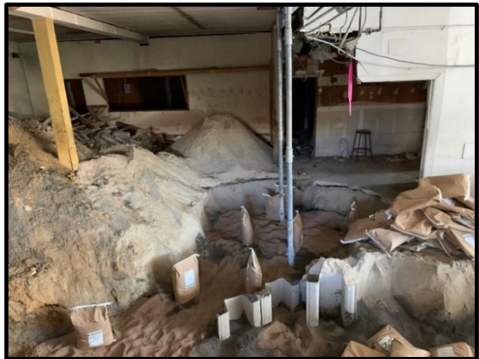
Figure 1: Provect-IR® Applied to Excavation
