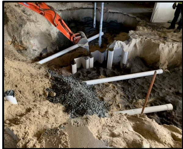
Figure 4: Soil Mixing and Injection Laterals
