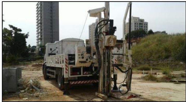
Provect-IR Applied via Direct Push Points
