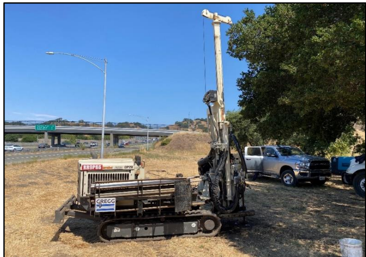
Figure 1: Provect-IR® Injection via Direct Push
